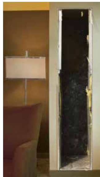
Remove internal components and trim cabinet edges.
