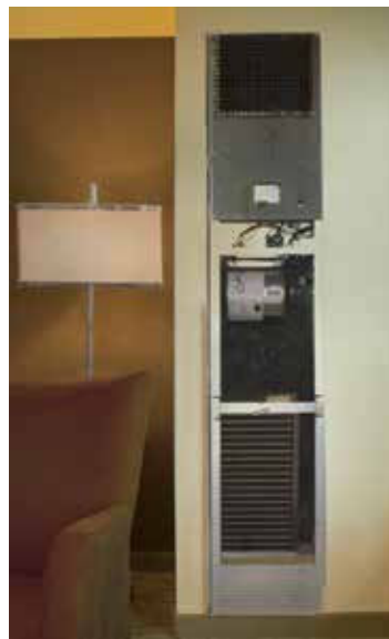
Remove surface components and trim drywall.
